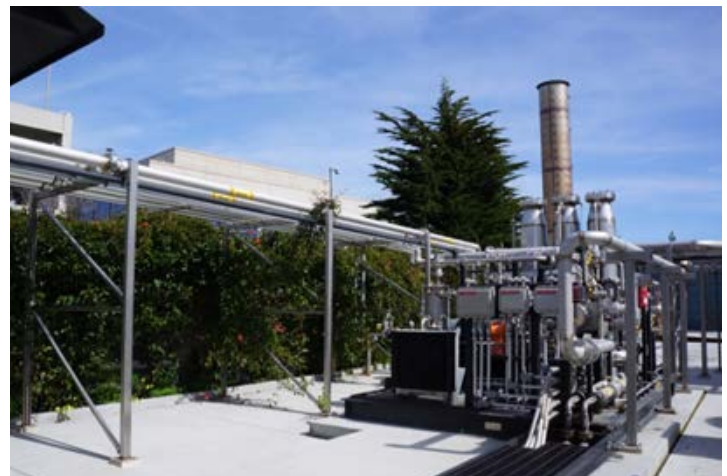
Biogas purification unit
