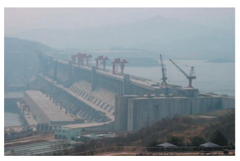
The project will be ended by the shiplift that will allow passenger boats up to 3000 tons to cross the dam in only 40 minutes. Today it takes 3 to 4 hours with the system of five ship locks for boats up to 10000 tons. This system of ship locks is the largest in the world: it is 280 m long and 34 m large, and it has been operating since June 2003.
